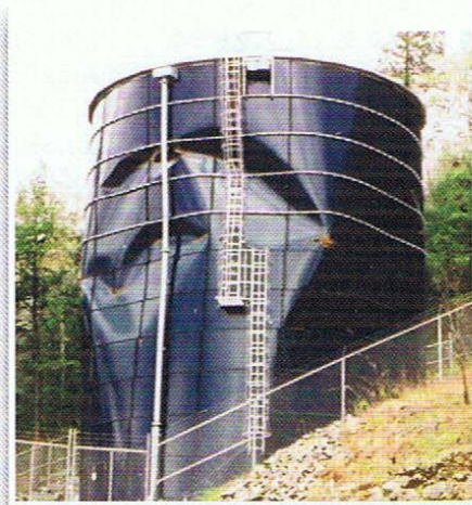
Figure 1. Buckled tank due to freezing.
