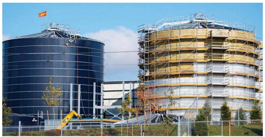
*In 2011, H2Flow Tanks & Systems Inc. erected a Permastore glass-fused-to-steel bolted tank at the original DOPF.*
